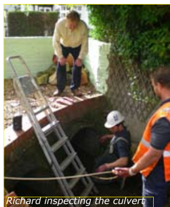
Richard inspecting the culvert
